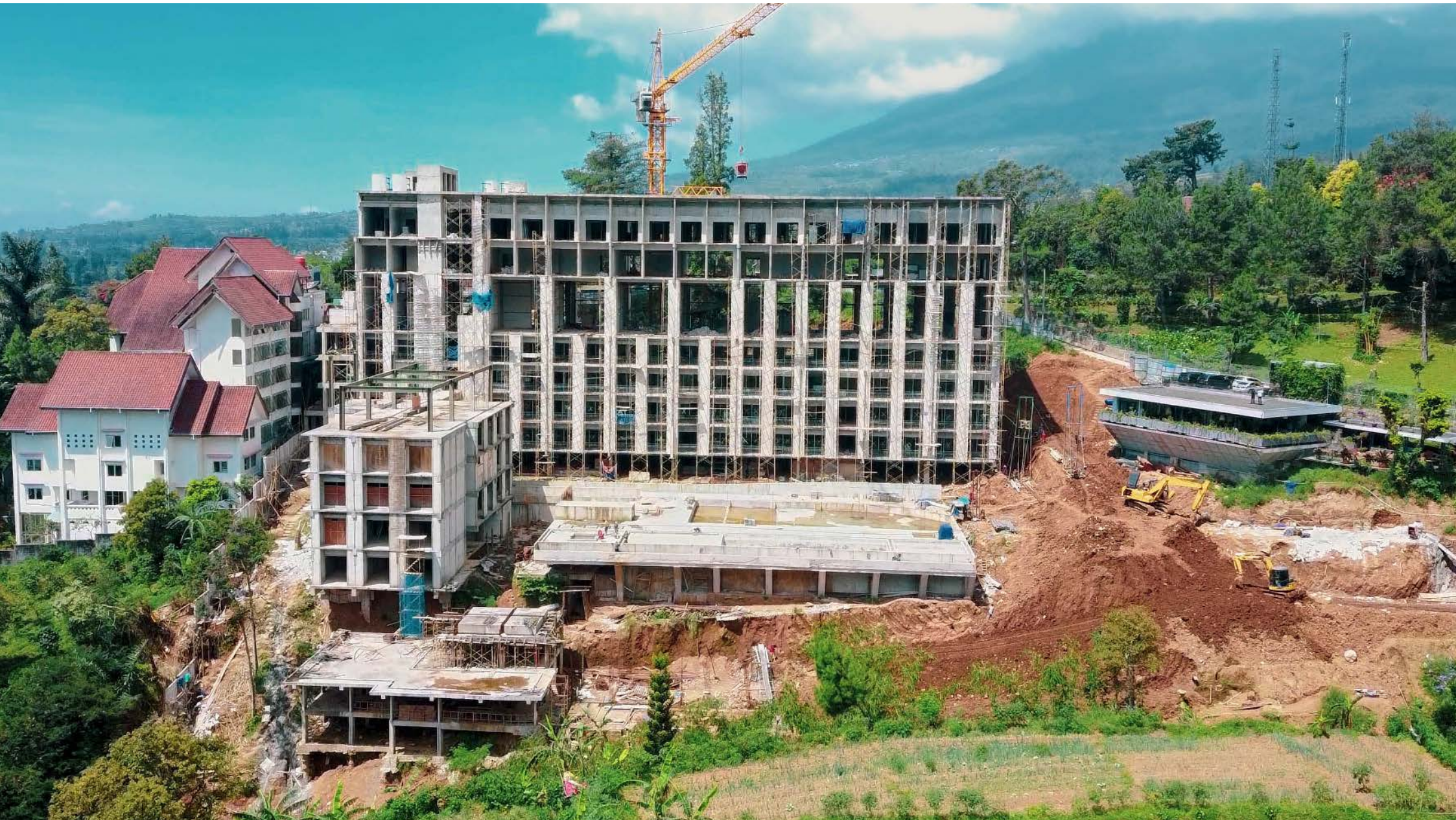
PROGRESS BY APRIL 2021
